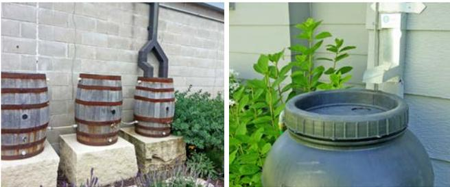
**Left:** Connected rain barrels capture more water for reuse. **Right:** A downspout is redirected into a rain barrel.
